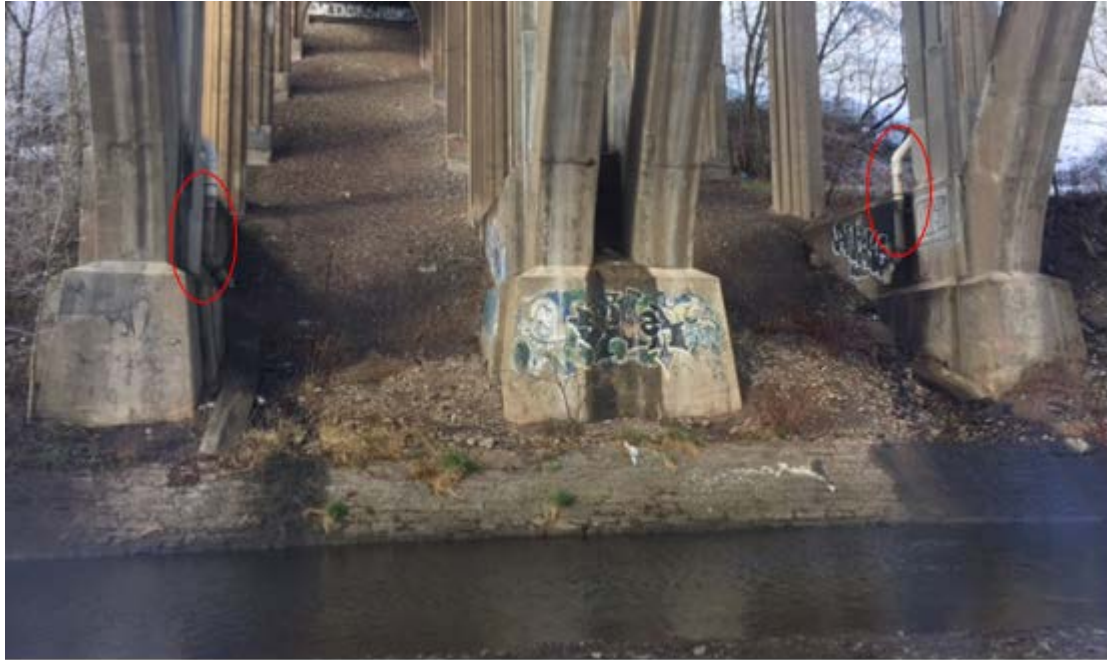
Figure 4.2 Drainage pipe from PennDOT bridge to NMR
