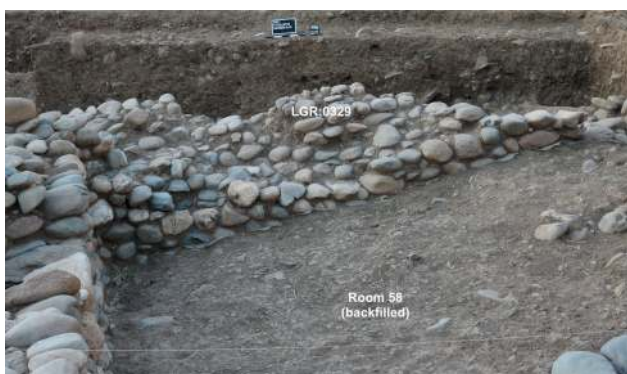
Fig. C14: Northern face of wall LGR:0329. Photo by Jens Rohde and Laura Tretow.
