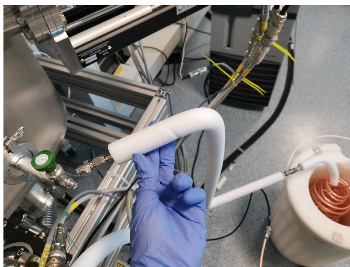
Figure 3-15: The backfill connections and the LN2 coil container.
