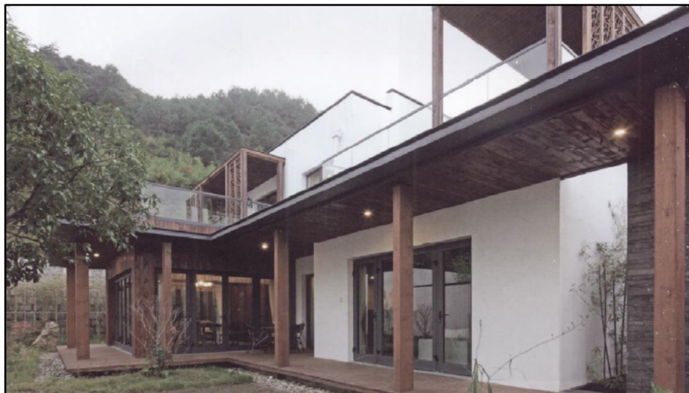
Figure 8.26. Huangshan No.1 mansion (source: Zhang, 2010, p.62).
