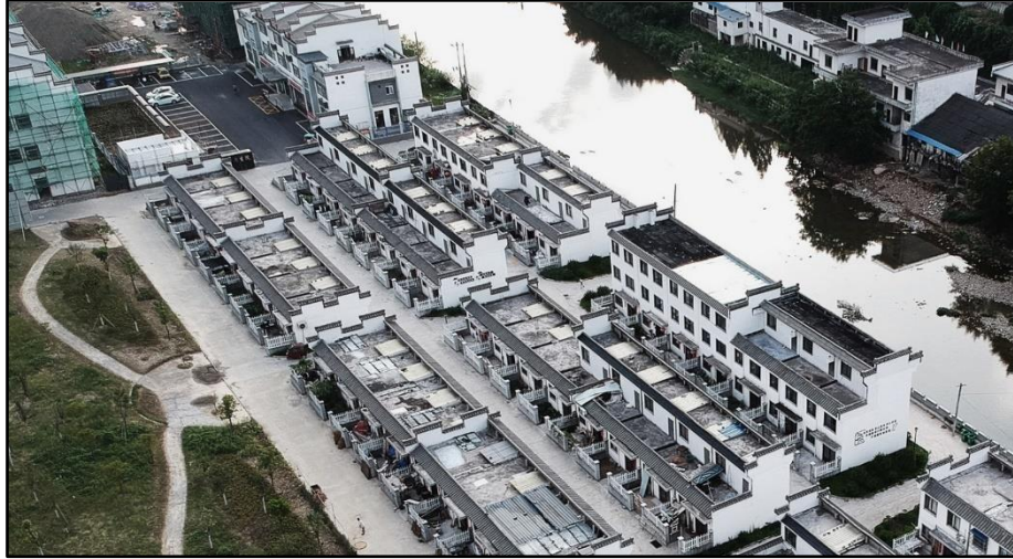
Figure 7.30. The compromise between Hui style and the regulatory constraint of per capita building areas (25 m 2 per people, one story or one and half stories) (source: Author).
