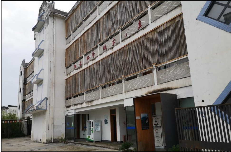
Figure 8.28. The hotel renovated by Deshui Company from a school, with low-tech bamboo pole curtain added (source: Author).
