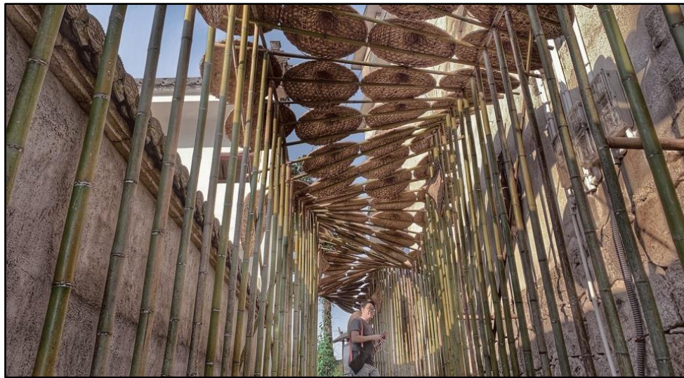
Figure 8.25. The bamboo ‘hat porch’ (source: Gooood, 2019. Available at: https://www.gooood.cn/the-bamboo-hat-porch-in-shang-village-china-rural-culture-d-r-c.htm ).
