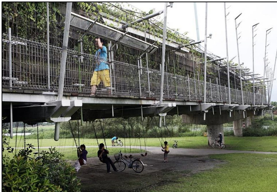
Figure 8.31. The Jinmei pedestrian bridge in Yilan (source: Youfang, 2010. Available at: https://www.archiposition.com/items/20180525100651 ).
