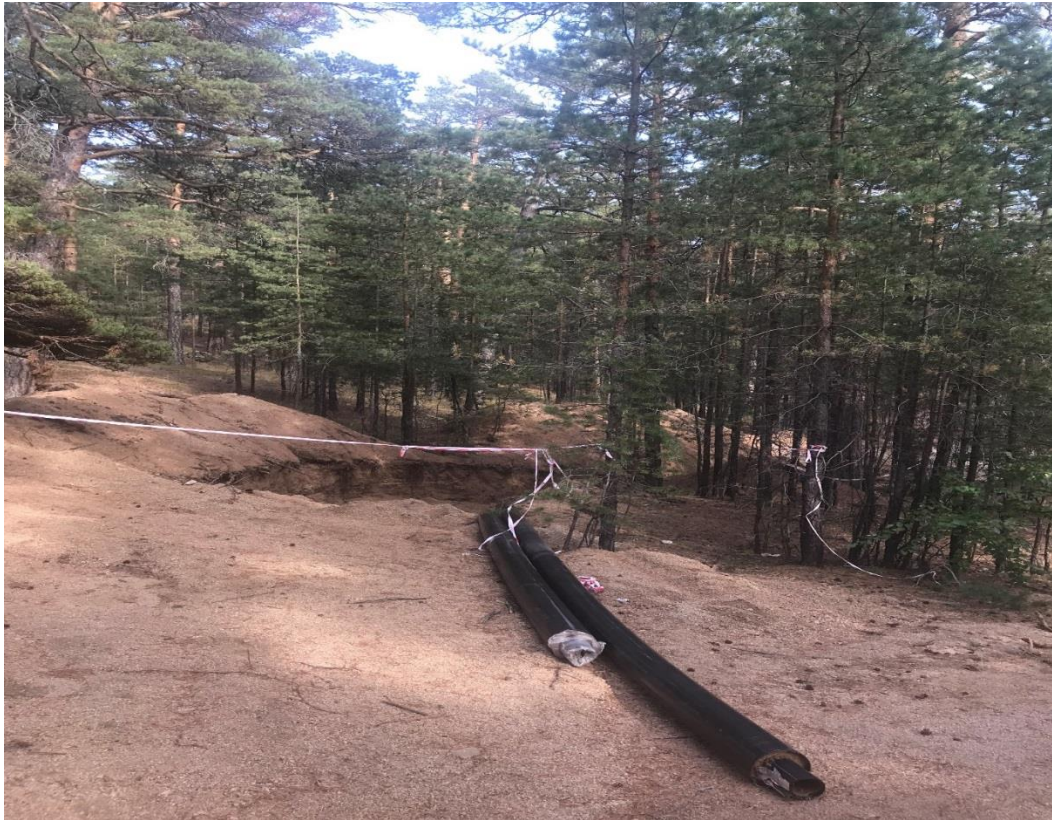
Figure 3. 9 Water supply construction in Burabay during summer 2019
