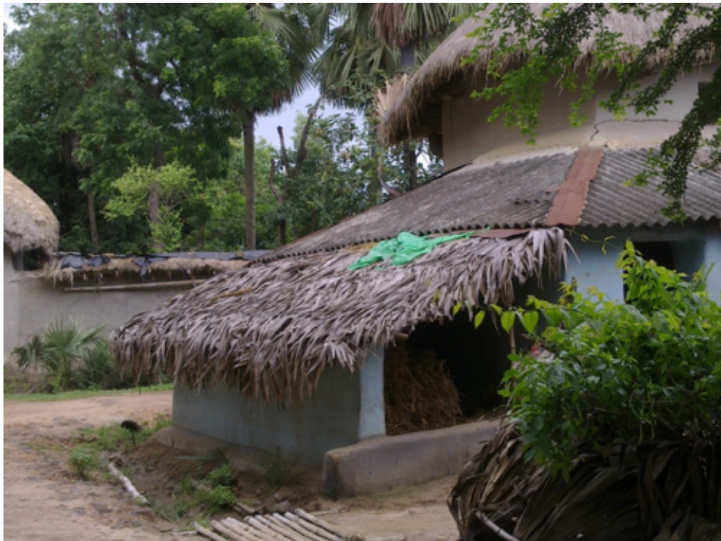
Figure 2.2: Typical house found in Kaligung and Pearson-Palli, made from bamboo or wood and mud.
