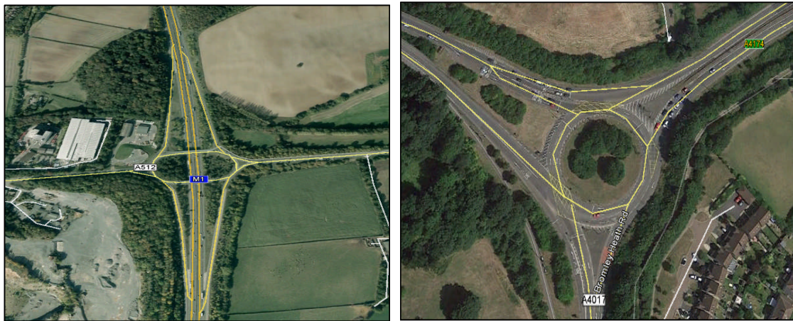
Figure 2-4 Aerial Photo of Four-Arm Grade-Separated Roundabout (Left), and Aerial Photo of Three-Arm At-Grade Roundabout (Right)
