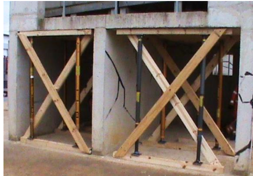
Figure 51 - Two post vertical shores
