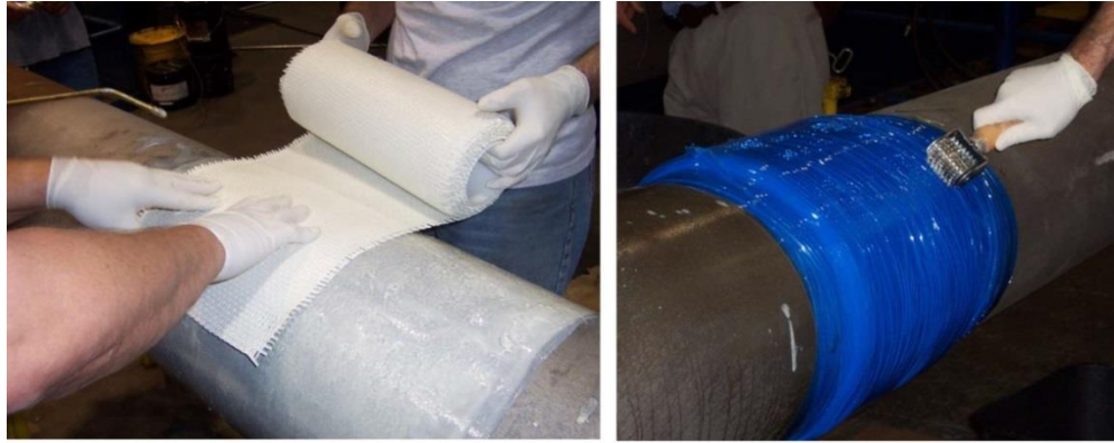
Figure 2-6, Installation of AquaWrap® on a corroded pipeline (Alexander 2005)
