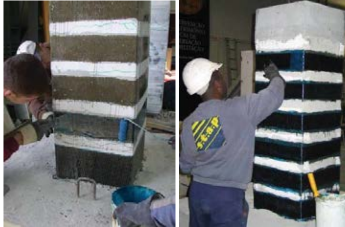
Figure 3: Pier reinforced with CFRP.
