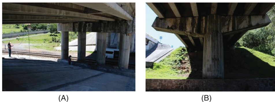
FIGURE 3 (A) Multi-column and (B) single column bridges in Mexico
