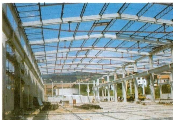
Figure 3. Industrial hall under construction
