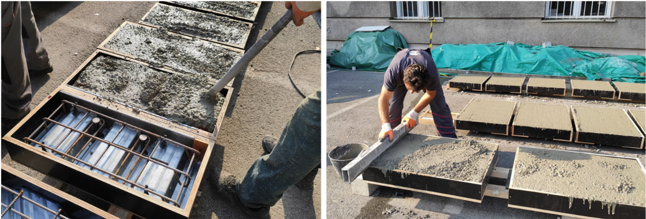
Figure 4.12: Concrete casting.
