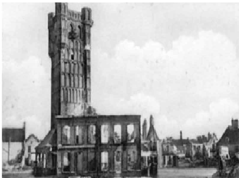
May 30th, 1940 - At the time of the seat of the city by the German troops (Operation Dynamo), the belfry is touched by a bomb flamer. All the frame disappears in the fire. It is finally dynamited on September 16th, 1944 by German at the time of their retirement
