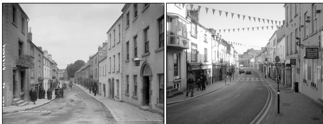
Figure 7.9 View of Lower John Street looking north; note the two-and three-storey houses and shops; Lawrence collection, Kilkenny, NLI, photograph L_ROY_10035; modern view, from the approximate same position, 18 Mar. 2016, Fergal Donoghue.
