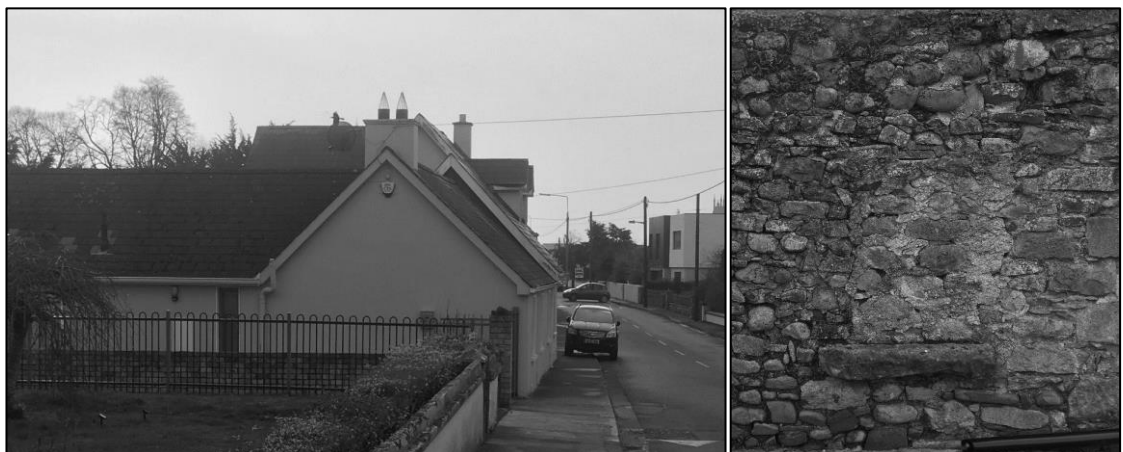
Figure 4.21 The only remaining house contemporary with the study period and a closed-up window opening in a rubble wall, also contemporary with the study period.
