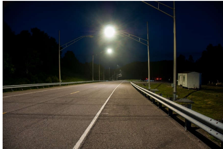
Figure 13. Smart Road Driving Facility.
