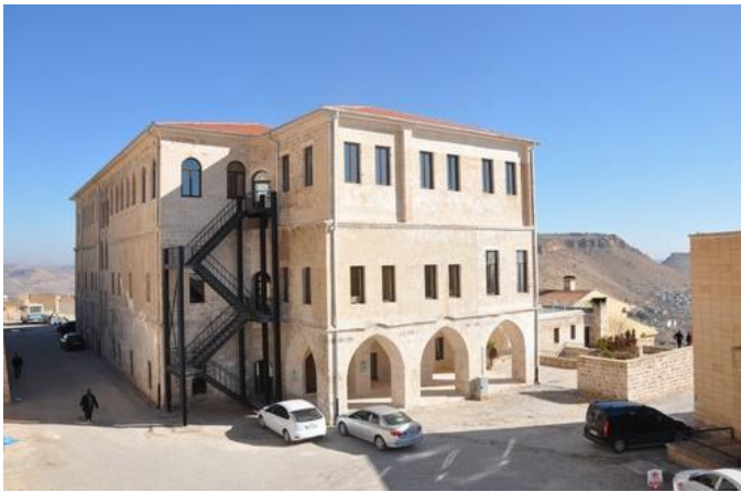
Fig. 13. Faculty building – a) Reconstruction of the second floor and roof during the period the building was restored in 2009 [40], b) Today's view
