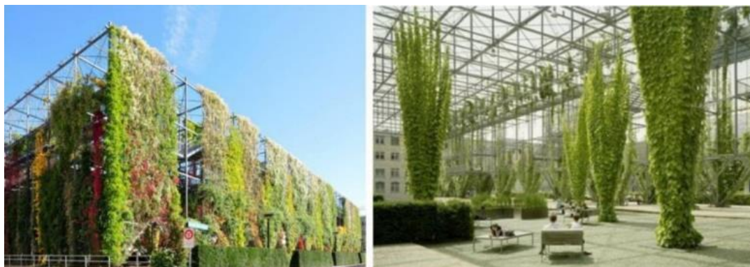
Figure 7: Grid and Wire – Rope system, MFO Park, Switzerland [25]
