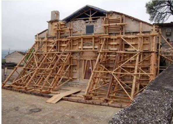
Figure 15: Propping of the buildings facades
