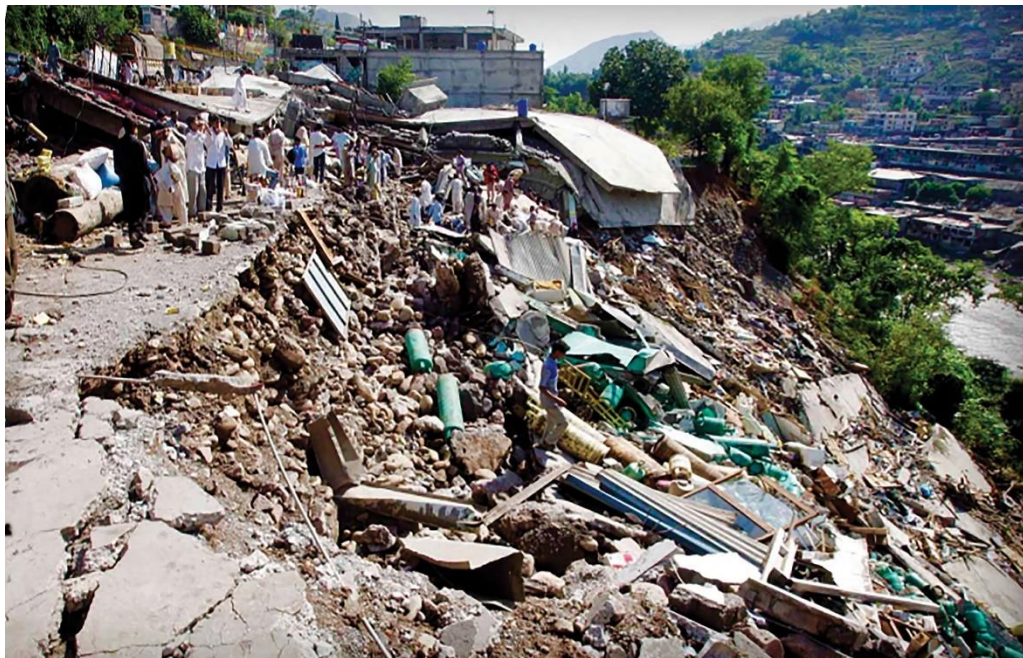
Figure 6. 2. Destruction of structures and hillslopes in Muzaffarabad, near the epicenter.
