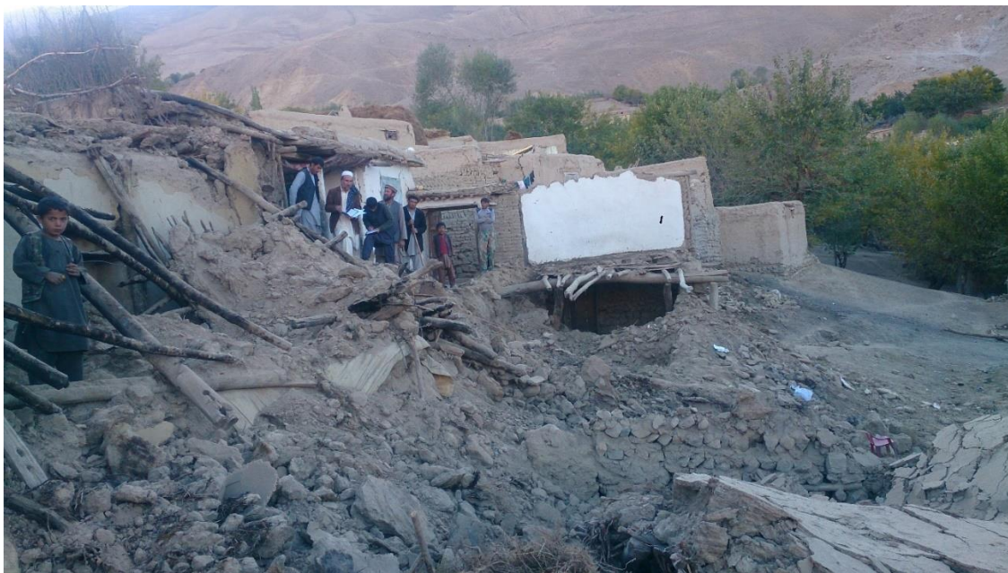
Damage to the countryside being assessed.
