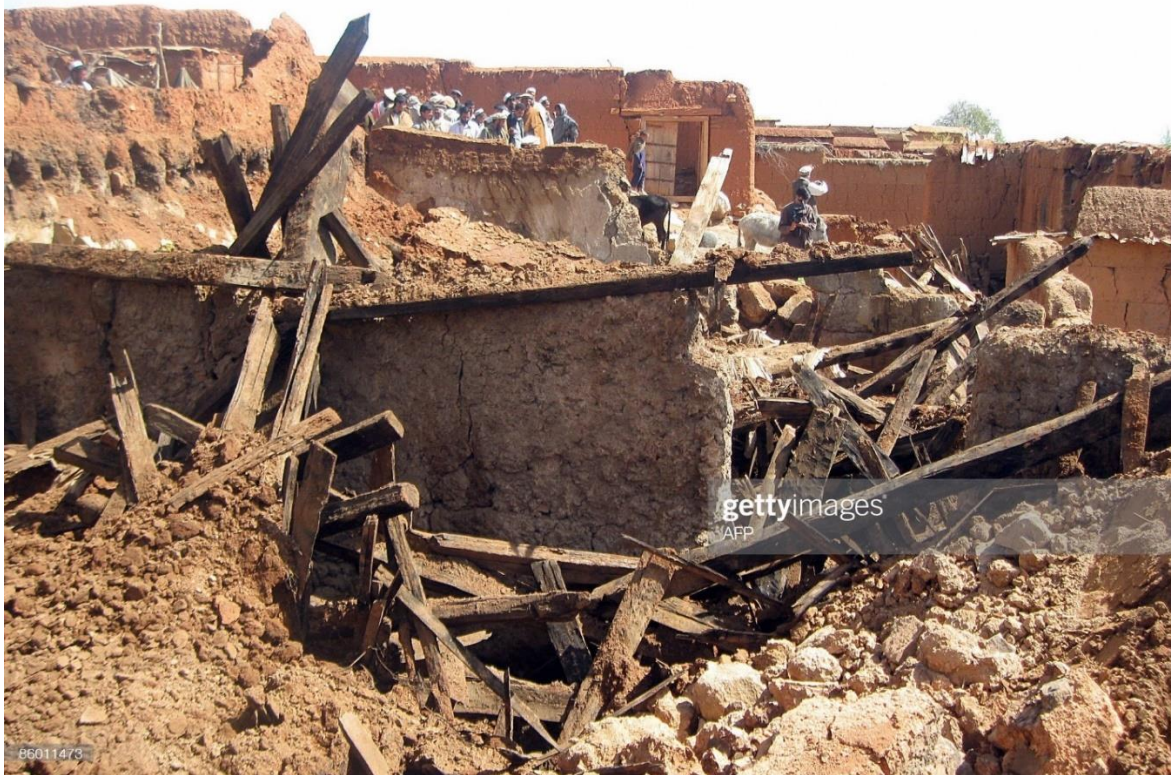
Extensive damages to an Afghan village in the eastern province of Nangarhar following 2015 Hindukush earthquake of Mw 7.5.
