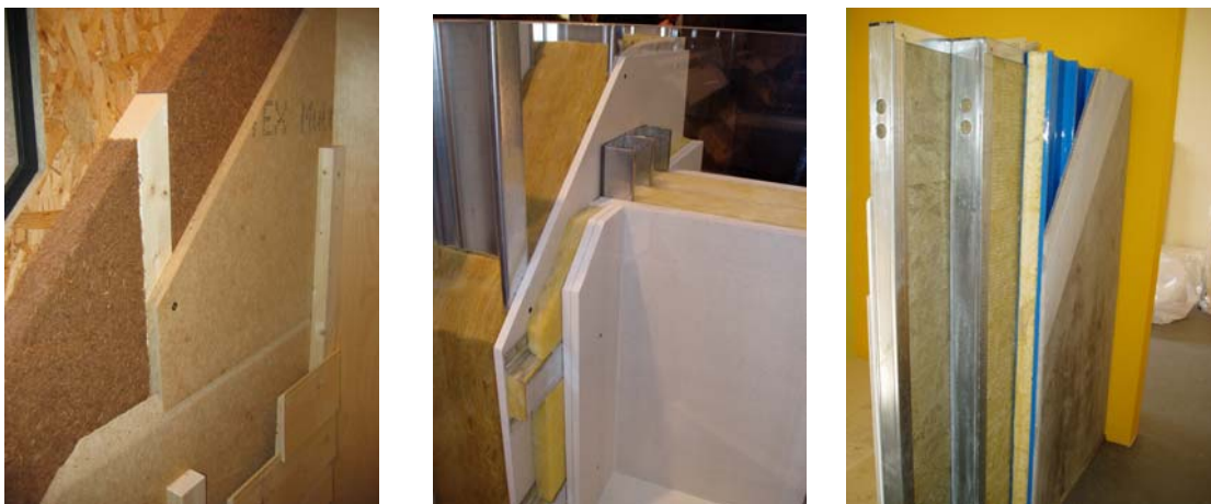
Figure 3: Examples of high-insulated envelope: the last one shows a mix of mineral and wood wool.
