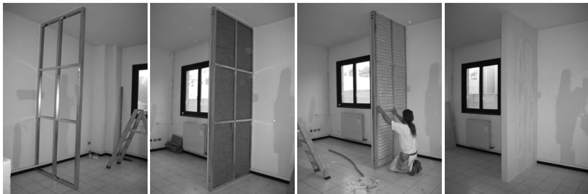
Figure 5: Sample of internal wall board, tested applying layers packaged in blankets containing PCM to provide artificial thermal inertia.
