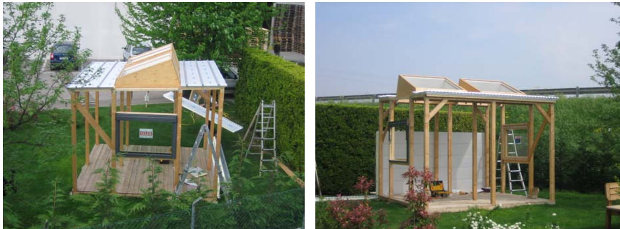
Figure 7 – The box built in Verona with roof windows containing PCM.
