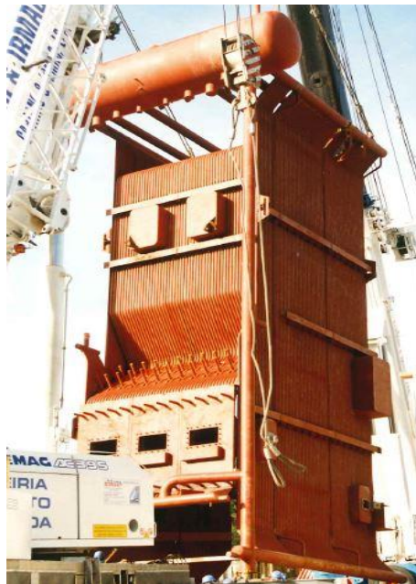
Figure 53: The grate-fired boiler.
