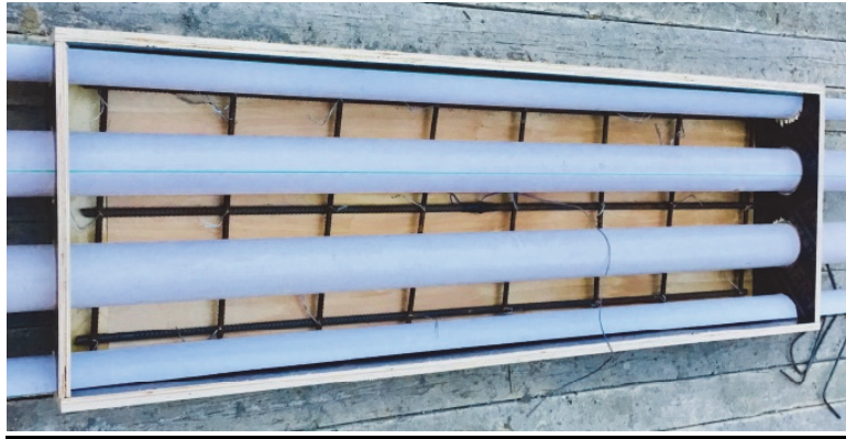
Figure 3: Mold preparation for the layered hollow core slab.
