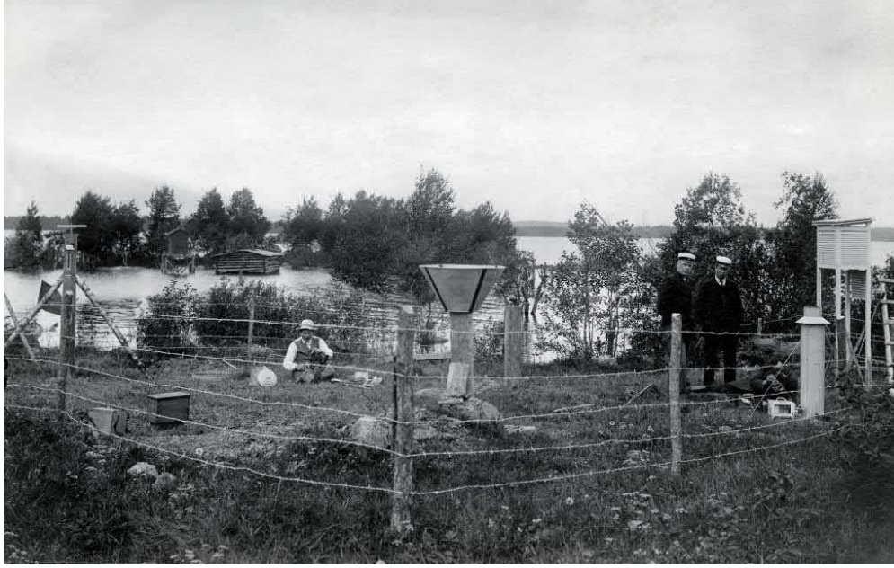
Figure 4.1: The village of Toppari had a weather station built for the evaporation measurements at Lake Pyhäjärvi, in Tampere (here pictured in 1912). Evaporation pans were installed in water near the shore, behind the peninsula visible in the picture. Photo: SYKE hydrological archive (Kuusisto 2008).
