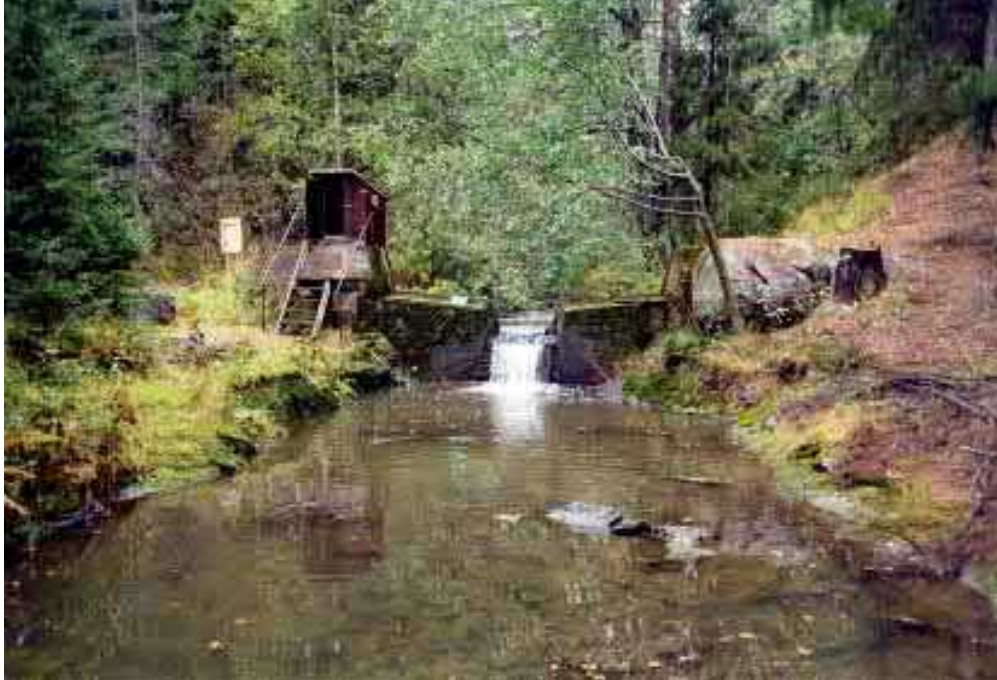
Figure 2.2: Niittyjoki measurement weir, built in 1958, standing near Kouvola, Finland. Weir can be used to determine the flow rate of a river. Catchment area of Niittyjoki is 29.7 km 2 and mean flow rate is 0.25 m 3 s -1 . Photo: Finnish Environment Institute (Kuusisto 2008).
