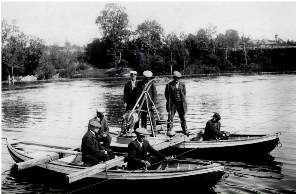
Figure 3.14: Flow rate measurements in Valkeakoski, 1913. Measurements are done with a paddle-type current meter. The current moves the paddles, and the rate of their turning can be translated into flow velocity with proper calibration coefficients. Measurements are done at several spots, and based on them the discharge rate of the river is discerned. Photograph: SYKE; Kuusisto, 2008.
