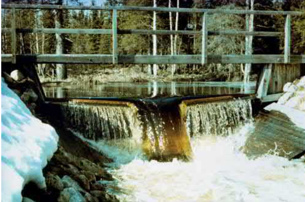
Figure 6.10: Melt water flowing through the Kotioja measurement weir in Ranua. The site was founded in 1976 for the investigation on the effects of forestry. Photo: SYKE (Kuusisto, 2008).
