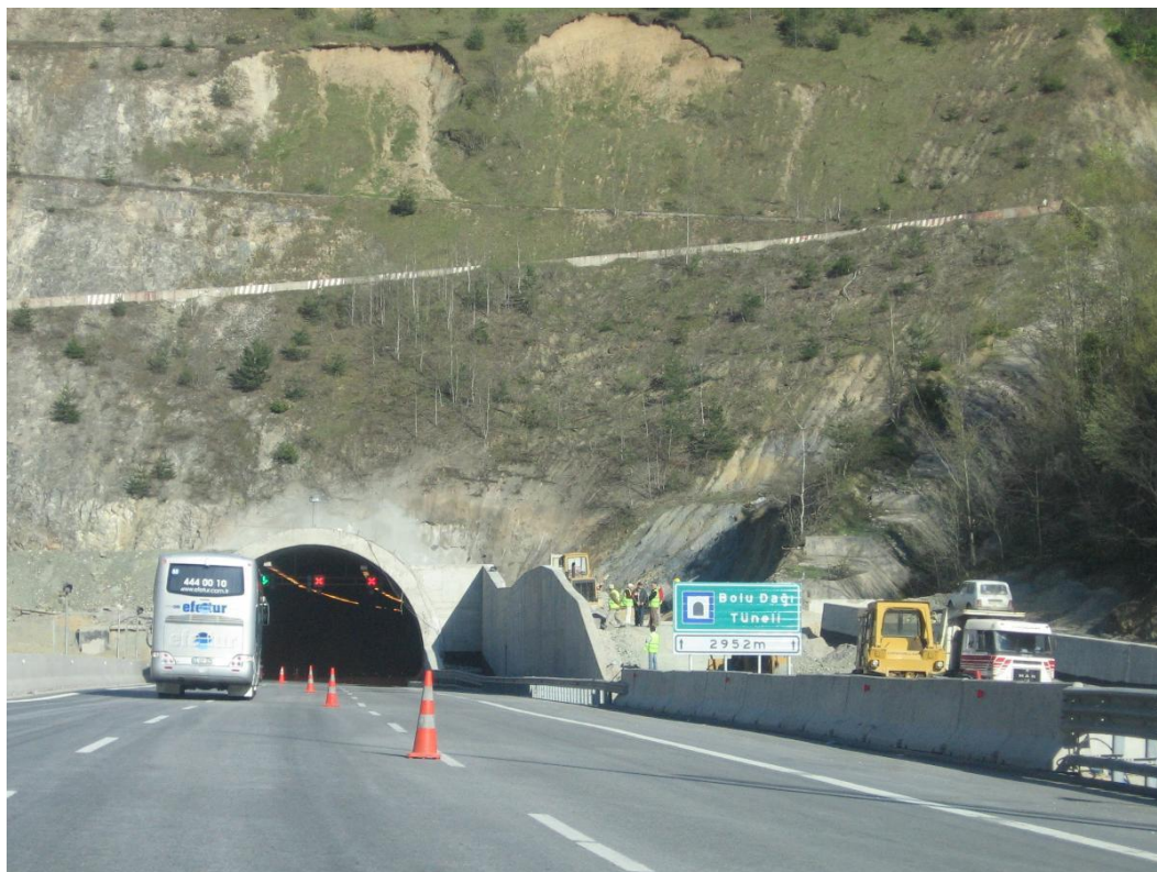
Figura 11 - Bolu Mountain Tunnel
