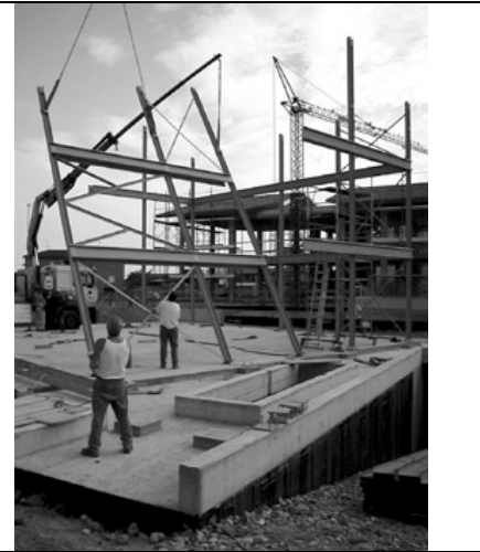
Figure 2: erecting one of the light portal frames.
