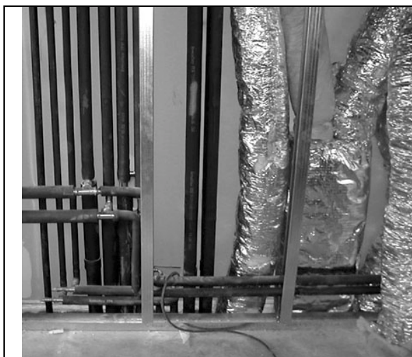
Figure 5: Str/En technologies allow for the easy flowing of ducts in the cavities of walls and floors.
