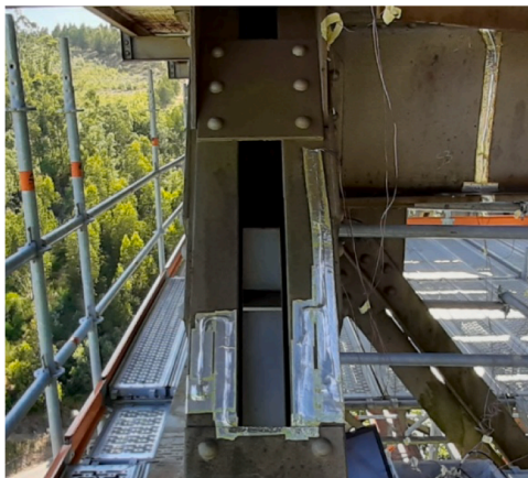
c) S9 and S10 (after the mechanical protection)
