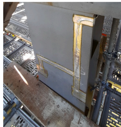
d) S12 and S13 (after the mechanical protection)
