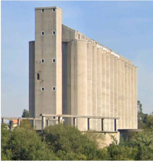
Fig. 8. Industrial building, view from the bridge over the Ave River.
