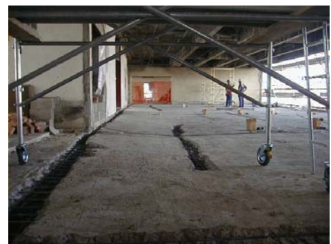
Fig. 4: Yield lines after concrete demolition
