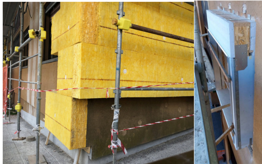
Figure 1. Image of the 25 cm thick external insulation; detail and photo of the window-wall node after the retrofit.
