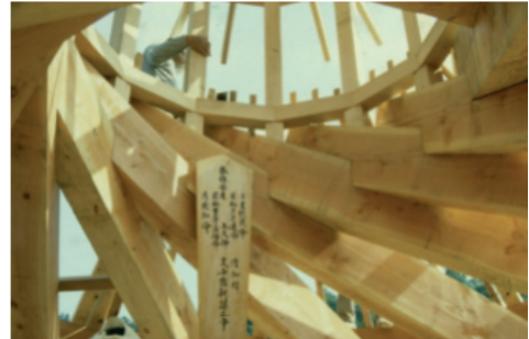
Figure 10. Seiya Exhibition Hall Roof Under Construction (Ishii 2004)
