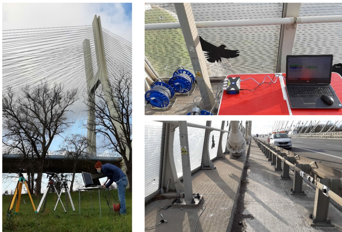
Fig. 4 Equipment layout at the ground measurement station (GMS; left), the deck measurement station at C7 (DMS; top right), and wired accelerometers mounted at C9 (bottom right)
