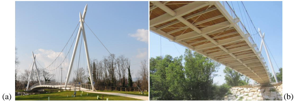
Figure 1. Seriate Footbridge: (a) overall view; (b) footbridge deck, detail of longitudinal and transverse beam.
