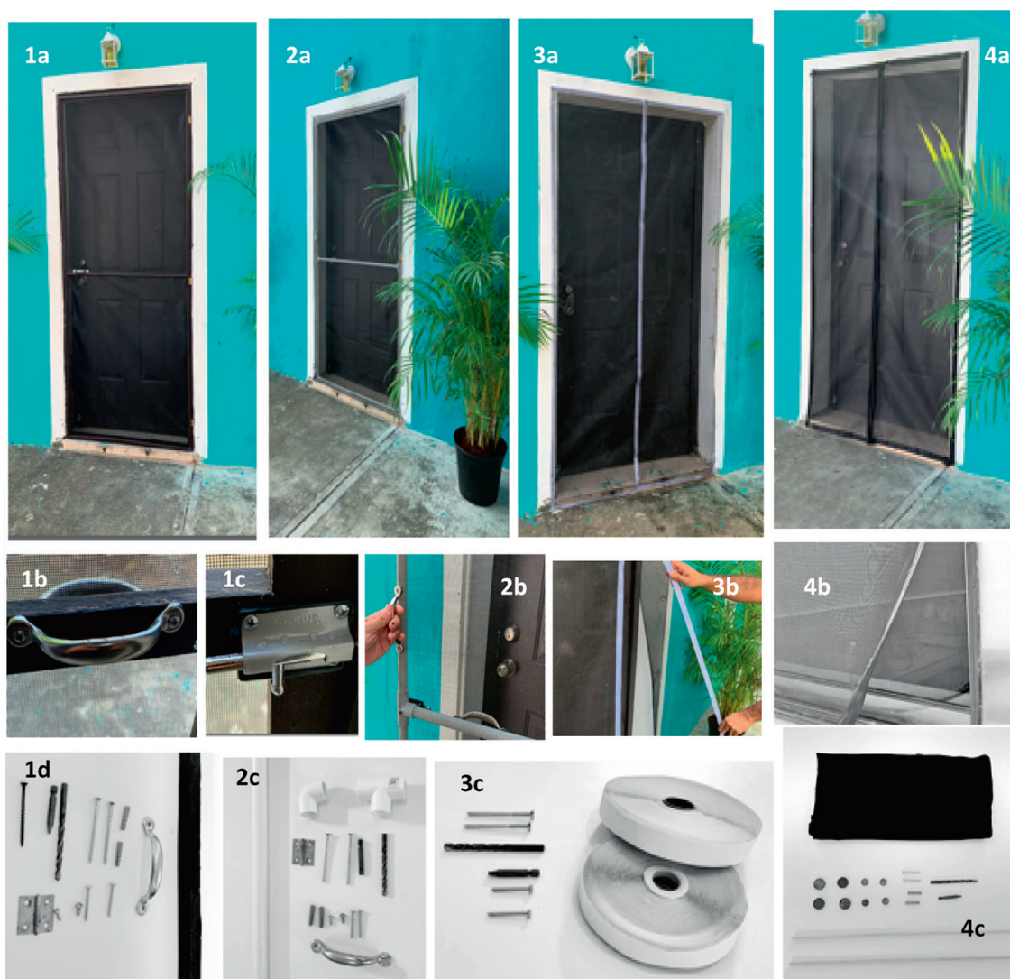
Figure 1. Different options and materials for the installation of house screening other than aluminium: (1a–1d) wood, (2a–2c) polyvinyl chloride plastic (PVC), (3a–3c) velcro and (4a–4c) magnets.
