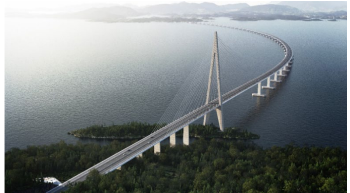
FIGURE 5: ILLUSTRATION OF CURVED FLOATING BRIDGE FOR BJØRNAFJORDEN, NORWAY. CREDIT: NORWEGIAN PUBLIC ROADS ADMINISTRATION.
