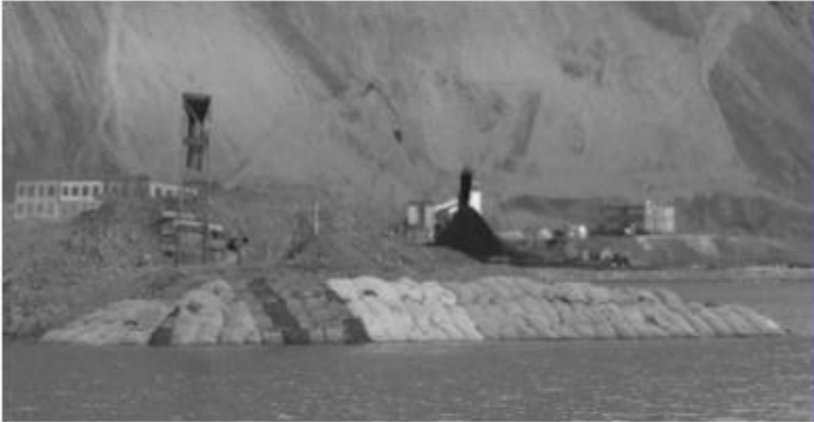
Figure 8. Use of “geo-bags” is tested for reducing erosion at Svea Mine, Spitsbergen (Reproduced from [31]).
