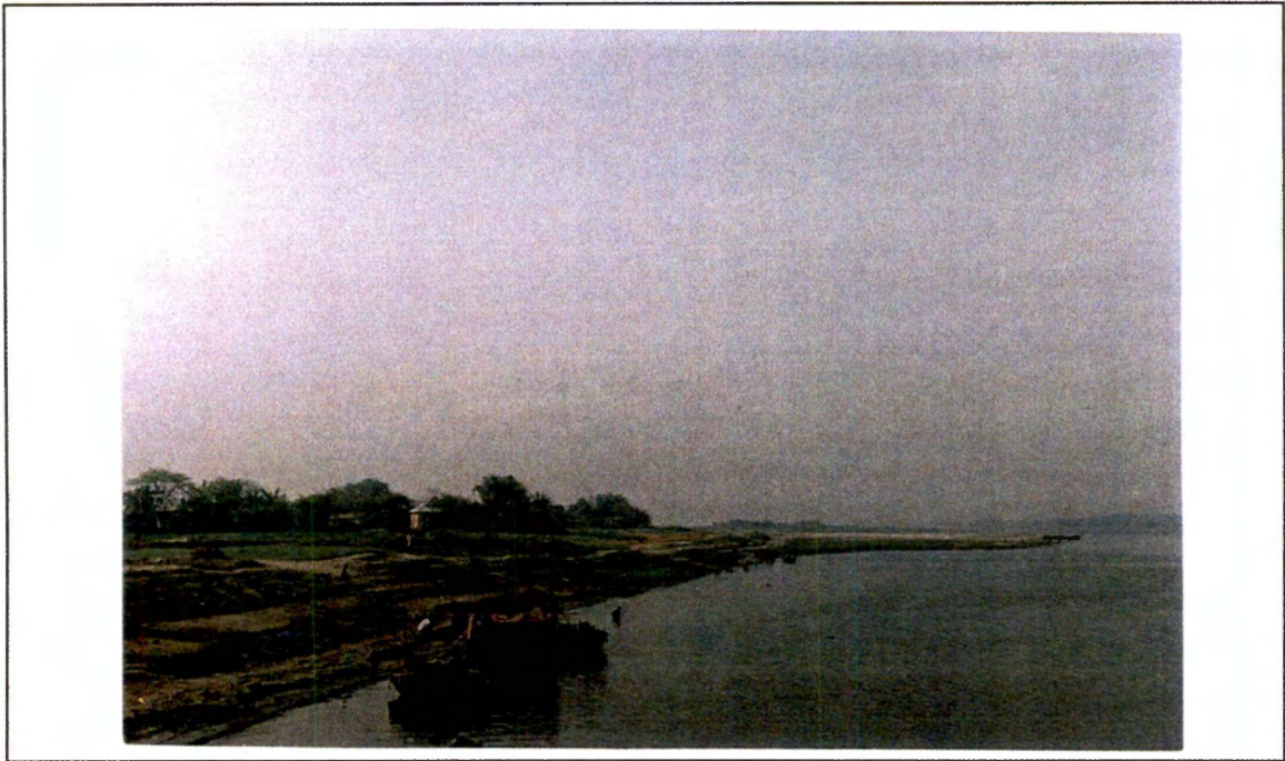
FIG 16: UNPROTECTED RIVER BANK AND VILLAGE
