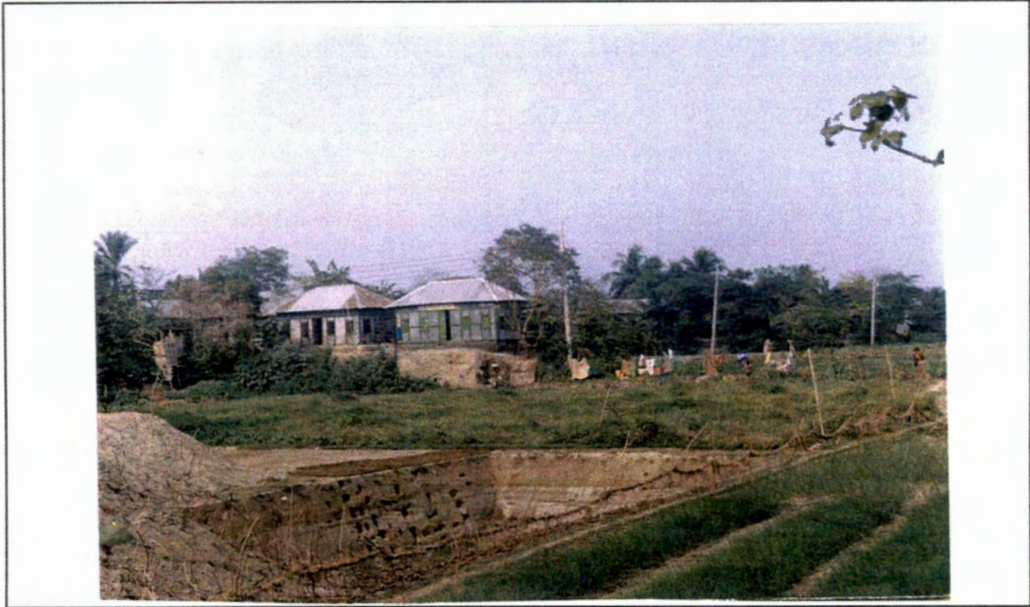
FIG 8: EXCAVATION OF SOIL FROM CROP FIELD
