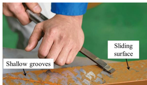
Figure 5.17 Photo of hand scraping. [58]
