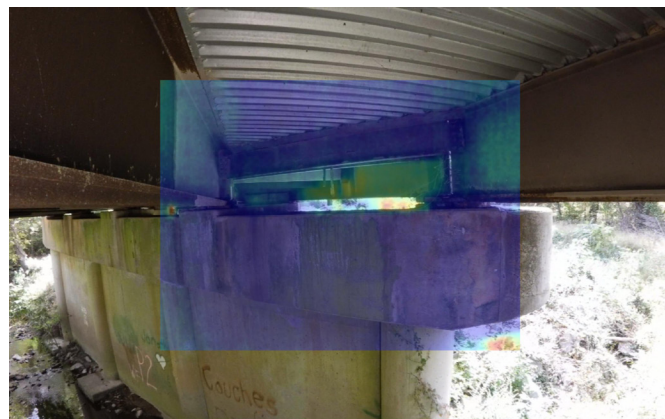
Fig. 6 Underside image of a deck taken from the Elios2 and overlaid with a semi-transparent thermal image
