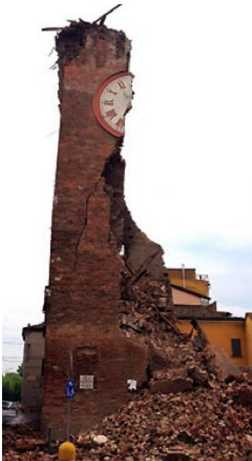
Figure 2: (a) Finale d'Emilia clock tower destroyed by the Emilia earthquake (2012, M_L = 5.8 ) and (b) San Bernardino bell tower, damaged by L'Aquila earthquake (2009, M_L = 5.9 ).
