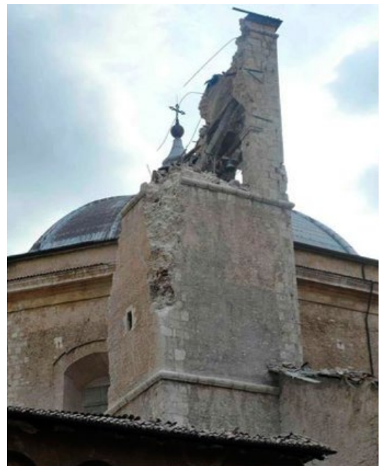
Figure 2: (a) Finale d'Emilia clock tower destroyed by the Emilia earthquake (2012, M_L = 5.8 ) and (b) San Bernardino bell tower, damaged by L'Aquila earthquake (2009, M_L = 5.9 ).
