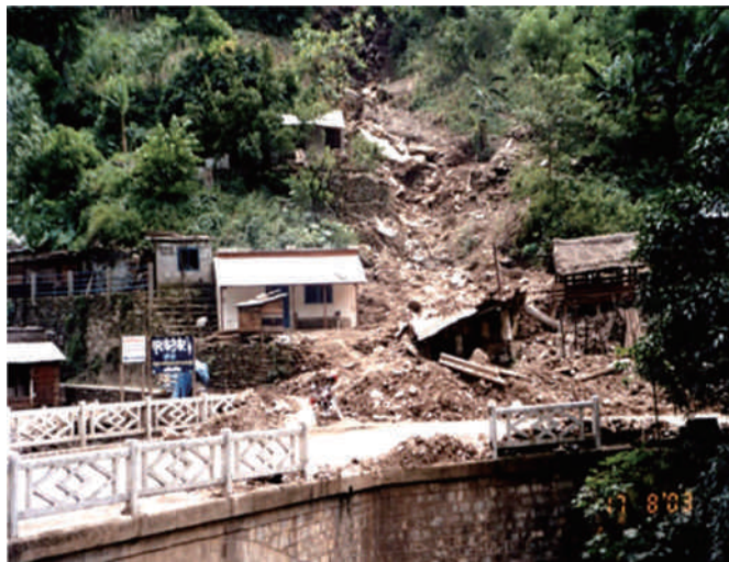
Fig. 10 : Photograph showing the damaged houses by the debris flow that occurred in 2003 at Jalbire
