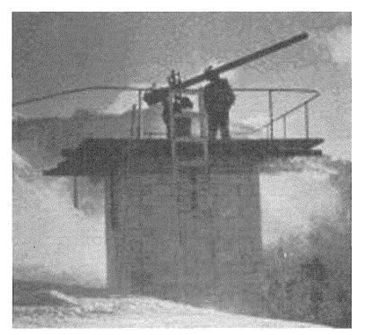
Figure 3 101mm Howitzer Recoilless Rifle used to artificially release avalanches Alyeska Resort photo, Girdwood, Alaska, USA
