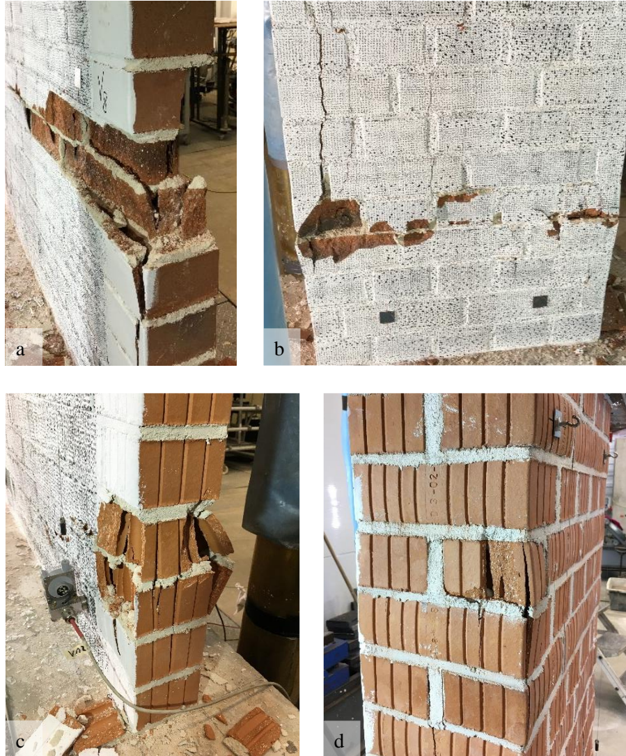
Fig. 4-13 Crack formation in the tests on reference walls (a: sw-sol-3, b: cb-sol-2, c: sw-perf-2, d: cb-perf-2)
