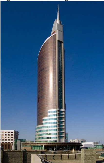
Figure 2. The building of the Ministry of Communications and Transport
