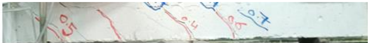
Figure 23. Crack pattern of spiral stirrups for spacing 40 mm
