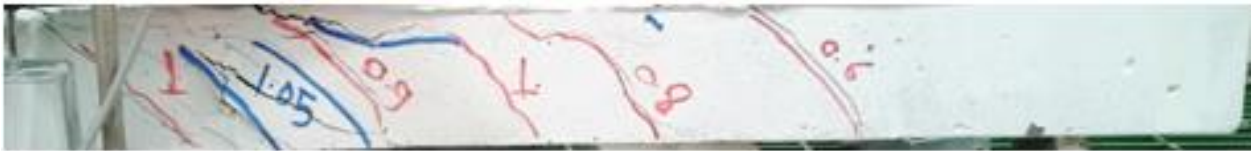
Figure 21. Crack pattern of spiral stirrups for spacing 20 mm
