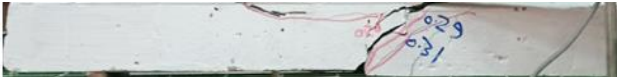
Figure 18. Crack pattern of closed stirrups for spacing 50 mm
