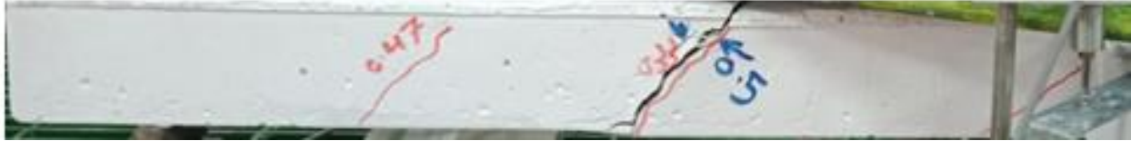
Figure 17. Crack pattern of closed stirrups for spacing 40 mm
