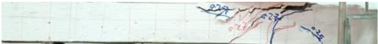
Figure 19. Crack pattern of closed stirrups for spacing 60 mm
