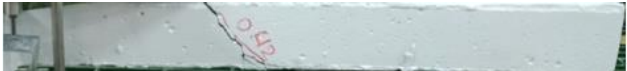
Figure 20. Crack pattern of closed stirrups for spacing 80 mm
