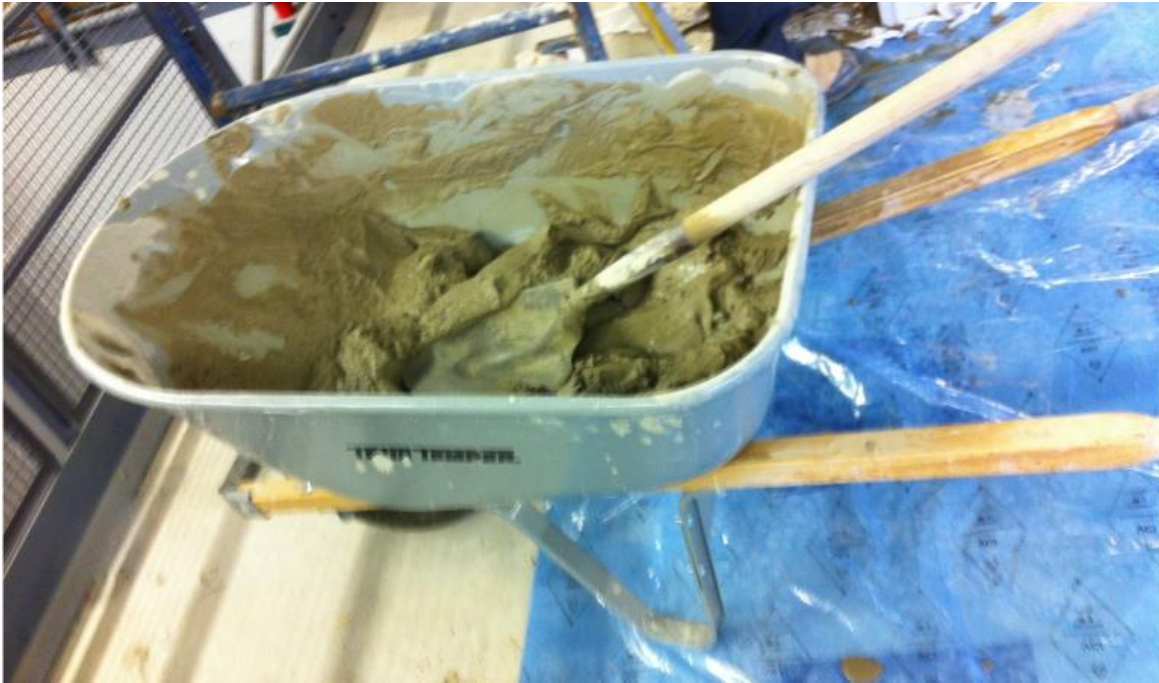
Figure A.2: Mortar mixed by hand in a wheelbarrow
