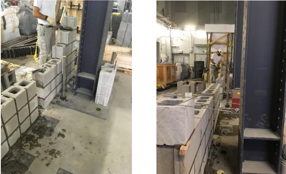
Figure B.4: Construction in a single line
