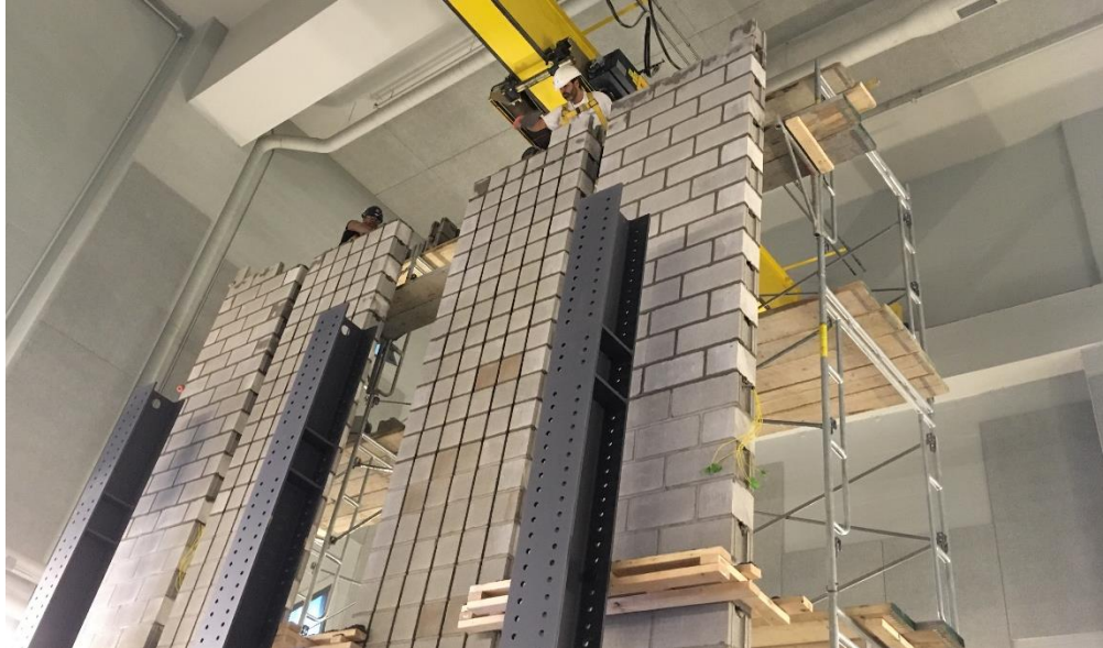
Figure B.8: Third stage of slender wall construction
