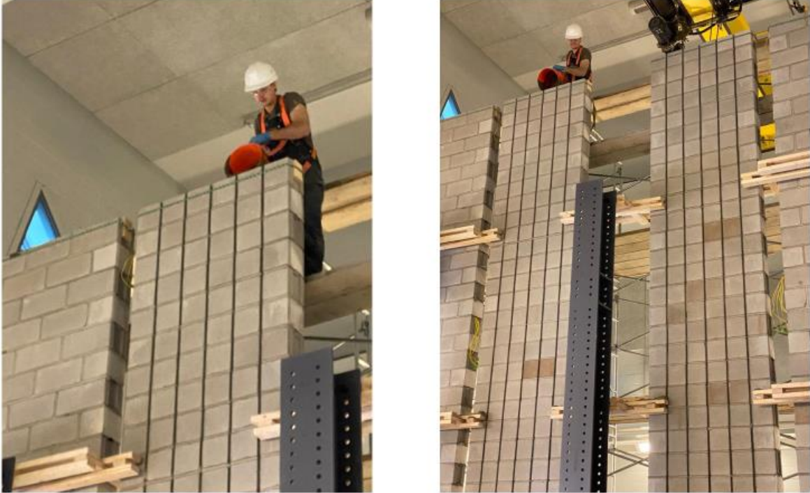
Figure B.14: Grouting third stage of slender masonry walls
