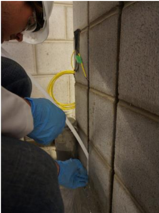
Figure A.13: Recessing of epoxy
