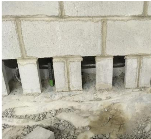
Figure B.11: Positioning of conventional reinforcing bars after the first stage of construction
