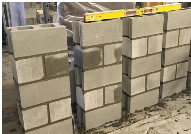
Figure 4.8: Masonry prisms made from conventional units during construction
