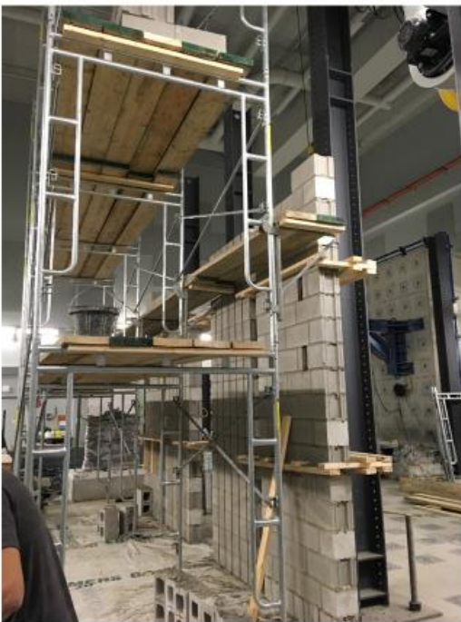
Figure B.6: Scaffolding for the second stage of wall construction
