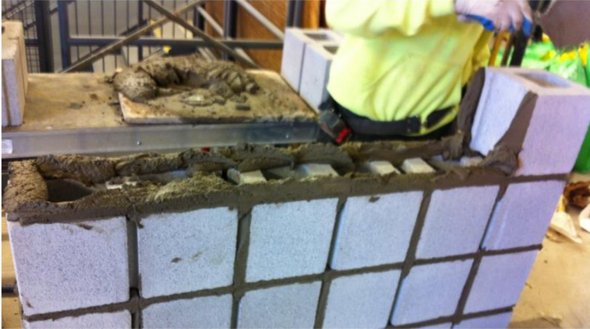
Figure A.4: Mortar filling vertical grooves of SRMUs during construction
