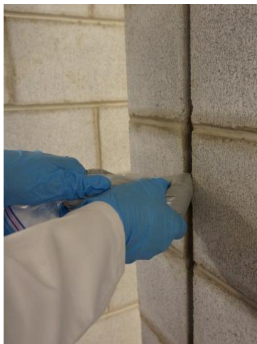
Figure A.11: Application of base layer of epoxy for NSM reinforcement
