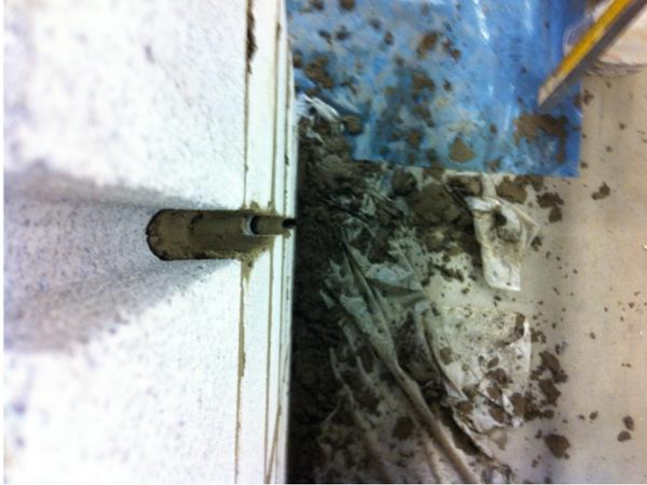
Figure A.6: Grooves in alignment and cleared of mortar
