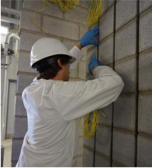
Figure A.12: Installation of NSM steel bars
