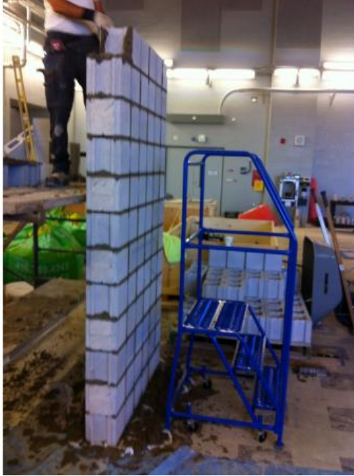
Figure A.7: Mason working on a freestanding platform
