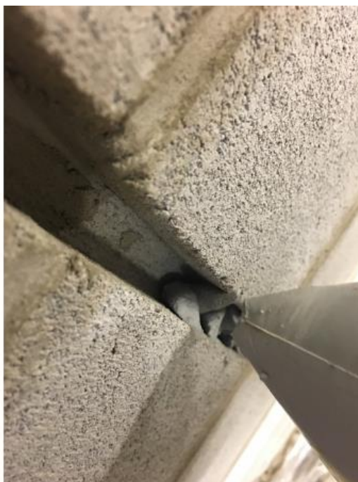
Figure A.11: Application of base layer of epoxy for NSM reinforcement
