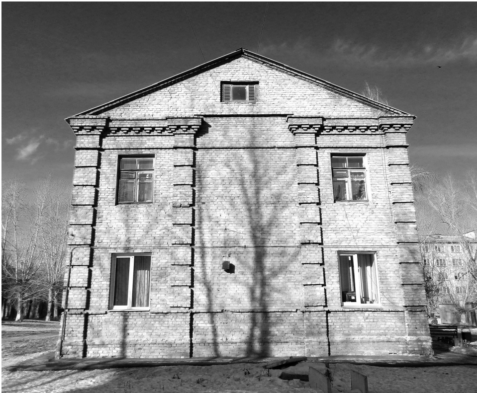
Figure 3. The photograph of historical building of former Military camp.
