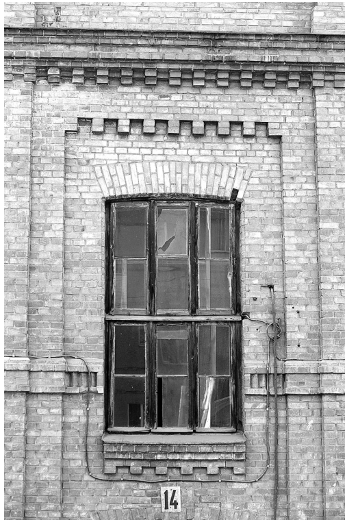
Figure 4. The photograph of historical building of former Military camp: a window.
