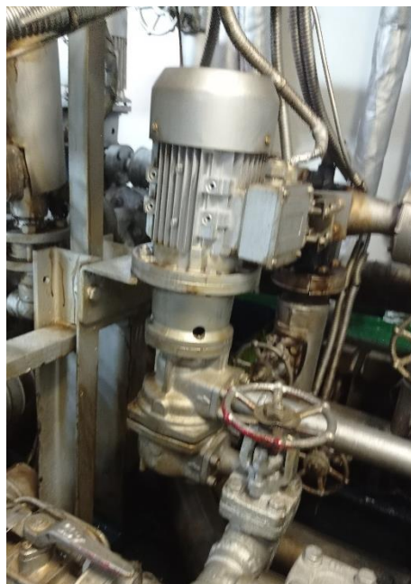
Figura 35 Bba Diesel
