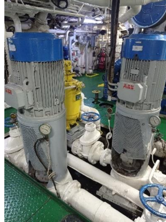
Figura 65 Bbas circ AT
