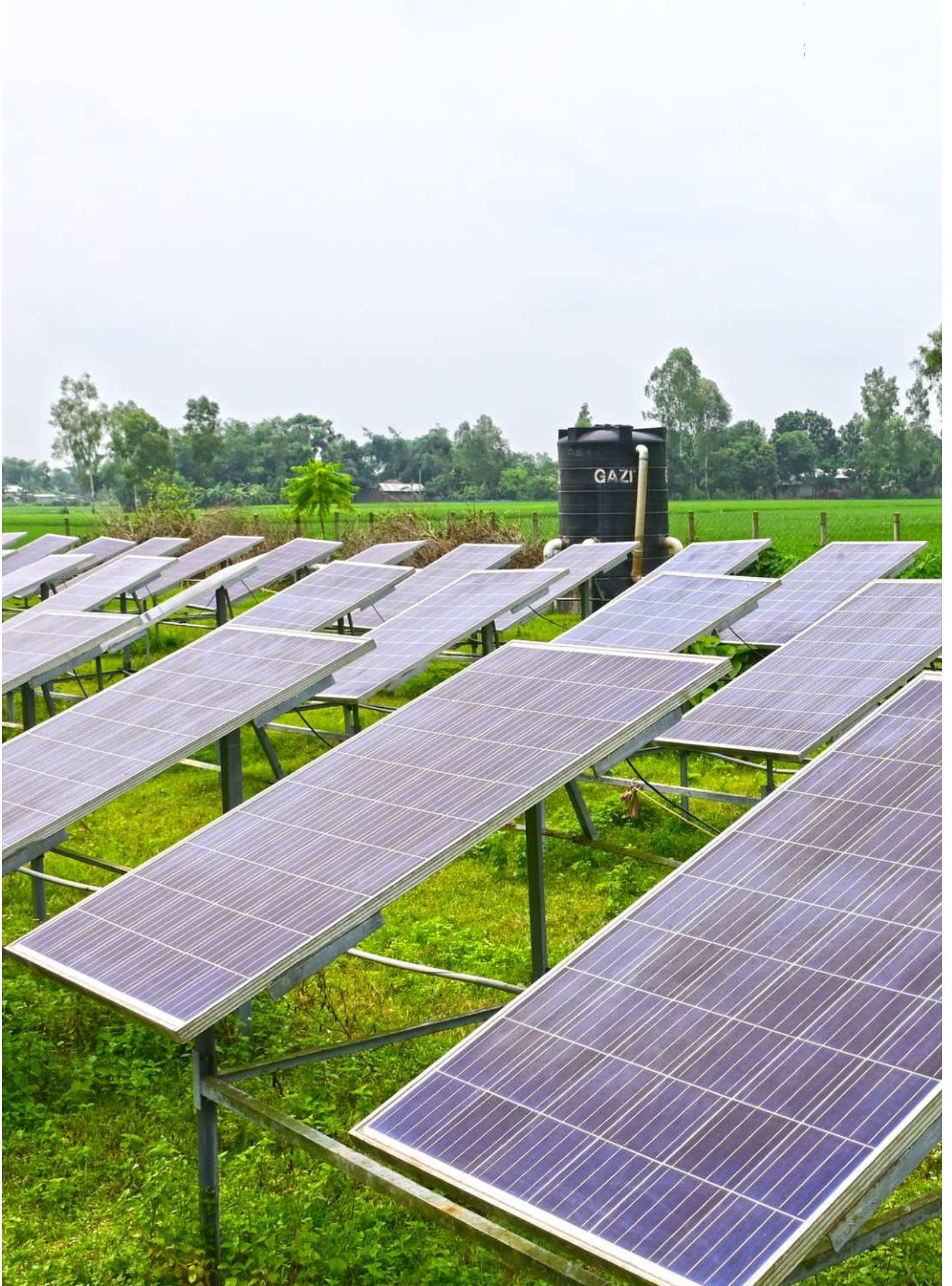
Solar panels in Bangladesh (photo: NGO Forum).
