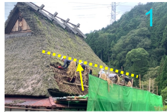
Removal of old thatch
