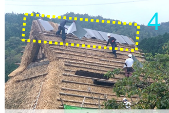
Placement of metal sheets
