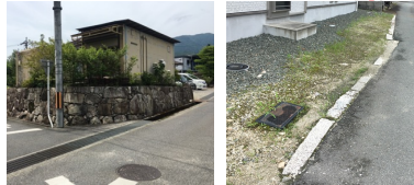
stone wall curb stone
